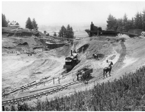
Construction of Reservoir 5 - June 4, 1910
